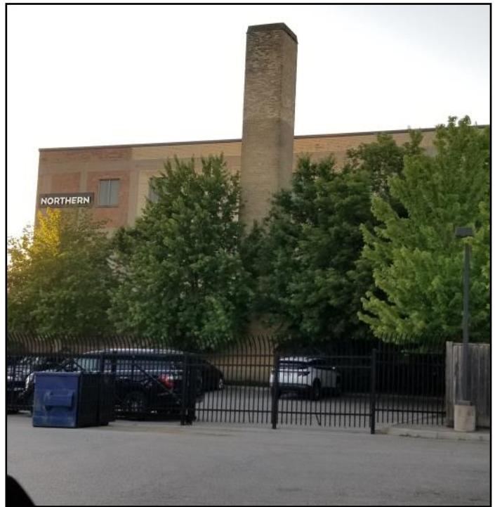
The view of the free-standing Phoenix chimney from a car parked in the Enterprise lot, looking northwest.
