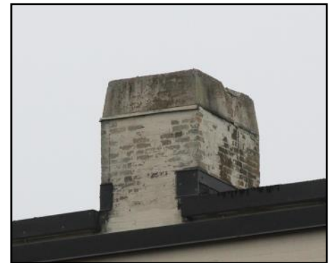
Close-up view of chimney at 388 Dundas.
