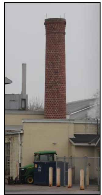
The Labatt's chimney viewed from the north.
