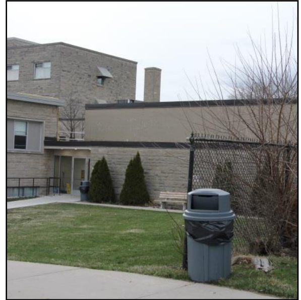
The chimney of the Wemple Building at King's College, showing the general area from which most monitoring was carried out. Barn Swallows nest under awnings over some of the windows.
