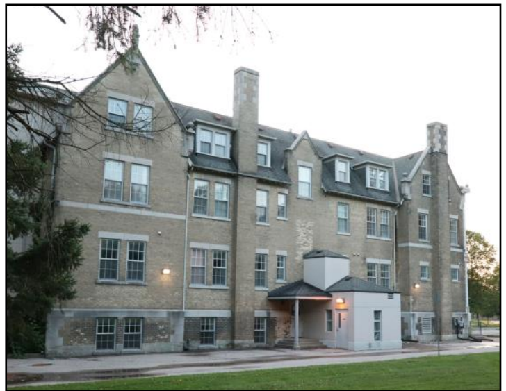
The rear (east side) of Kingsway Academy, south chimney on left, north chimney on right.
