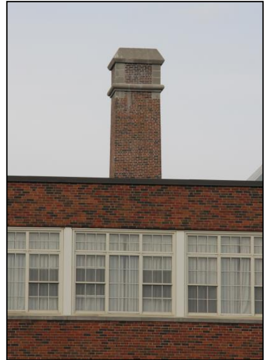
The South Collegiate chimney viewed from the front (north side of the building).
